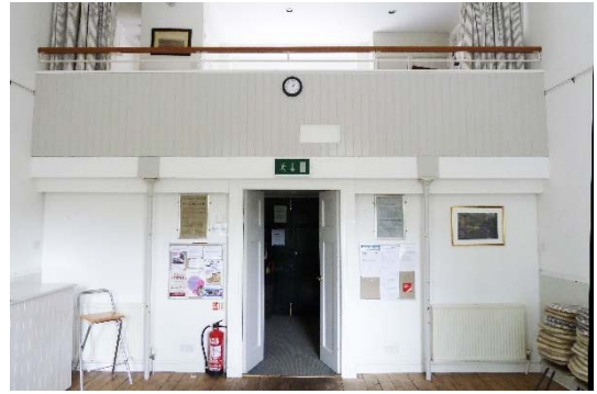
Blockley Little Village Hall – historic balcony
