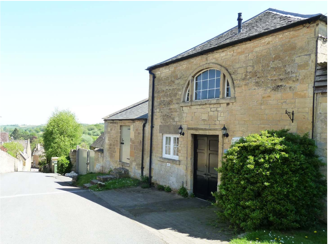
Blockley's Little Village Hall – external view of listed building
